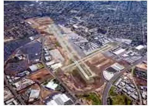
Photo by Fred Emmert AirViews.com Photo taken 10-Dec-2014 looking northeast.
